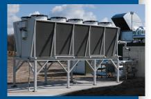
▲ The Güntner condenser GVD, specifically developed for the energy industry, cools the working fluid used in the ORC process.
