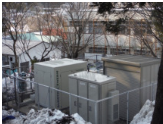
Figure 7: ORC Installation Central Japan
