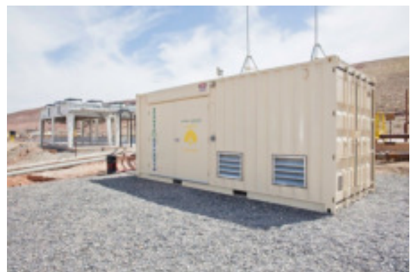
Figure 4: The ORC at Florida Canyon Mine in Nevada
