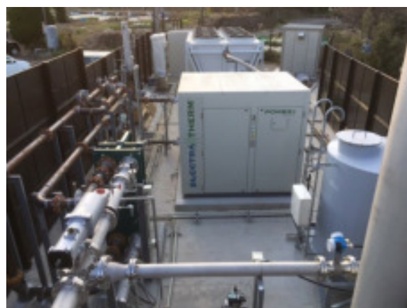
Figure 6: ORC Installation at Beppu Japan
