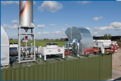
▲ Unit on the left: The Güntner GFH drycooler serves as oil-mixture cooler; unit on the right: The Güntner GFH drycooler serves as emergency cooler that can be used e. g. during maintenance work on the block heating station.
