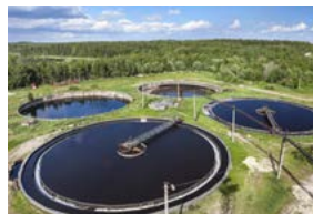
Waste Water Treatment
